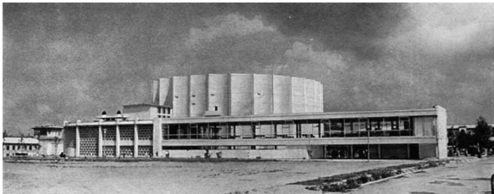
29. Panoramic cinema in Tashkent; architects - Vladimir Berezin, Sergo Sutyagin, Yuri Khaldeev, Dmitry Shuvaev, 1964
