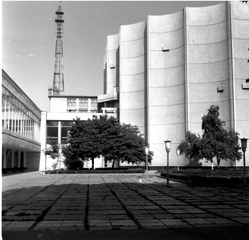
28. Panoramic cinema in Tashkent; architects - Vladimir Berezin, Sergo Sutyagin, Yuri Khaldeev, Dmitry Shuvaev, 1964
